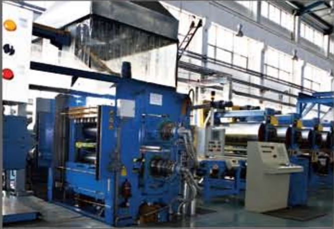
The innerliner production line made by Troester, Germany.
